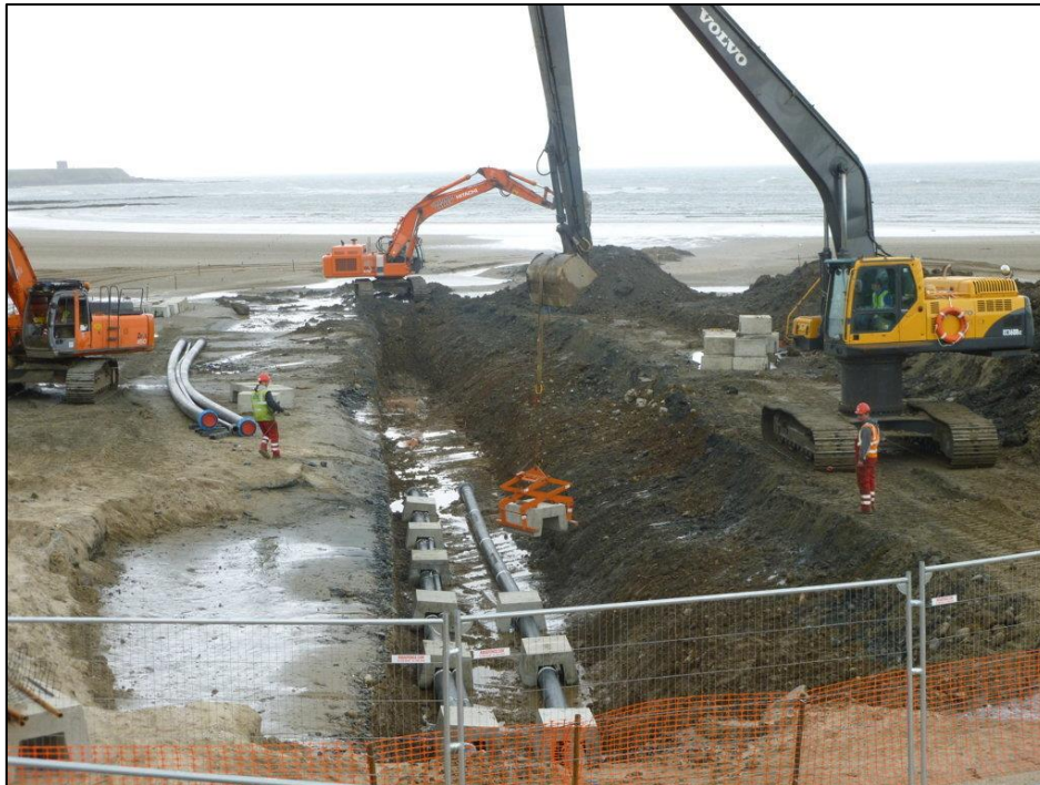
Figure 15: Example of an open-cut trench (source: EirGrid)
