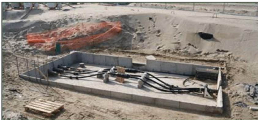
Figure 7: Landfall chamber under construction (RTE)
